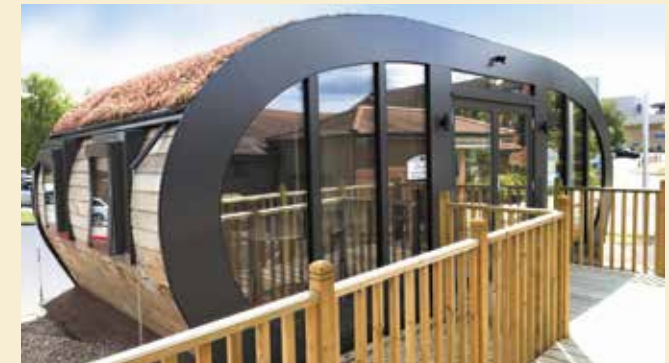
NEW MODULAR ECO BUILDING
